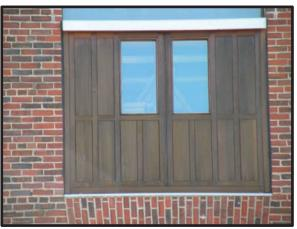
Figure 7.4. Second floor, teak fenestration unit, north elevation.
