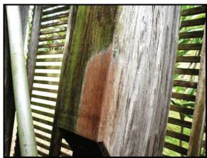
**Figure 2.4.** Example of biological growth and weathered patina, both of which can be removed through careful cleaning.
