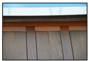
**Figure 7.6.** The relatively protected teak just below the flashing has retained a much lighter color after treatment than the more exposed teak.
