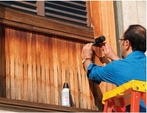
FIGURE 4.25 Project team conducting a visual condition survey of the window wall assemblies. Image:
