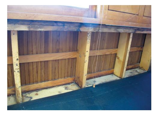
of the units. Minor damage was noted in the upper portions of the framing, such as at the stops for the sliding windows and louvers. The area of damage also corresponds to an area exhibiting significant moisture staining along the base of the wall framing.
