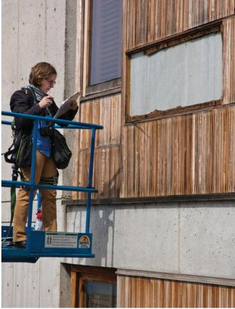
Salk maintenance staff have been diligent about reinstalling fallen boards or replacing in-kind at areas in public view or easily accessible by ladder or lift.
