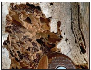
**Figure 2.5.** Example of typical drywood termite galleries discovered after breaking through a thin shell of sound-looking wood. Note the collection of frass. Awl handle in foreground is shown for scale.
