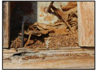
**Figure 2.6.** Frass found behind a teak slat removed for specimen analysis, study tower 10, NU7C.
