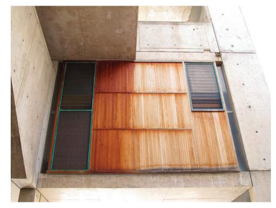
covered by the roof, such as the lower-level window walls of the studies that face the gardens, there can be a dramatic shift in the red appearance across the exterior face of a single window wall as it weathers away.
