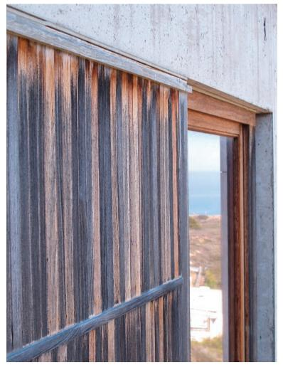
North wing office, north-facing window, sixth floor (NO6A). The teak exhibits minimal erosion, and the horizontal drips still overlap the tops of the vertical T&G boards. Image: J. Paul Getty Trust.
