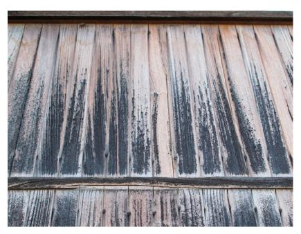
Detail view of a west-facing window in the northern west office wing (NO6J). The fungal biofilm presents as a black, sooty material deposited on the surface of the teak or in the cracks.
