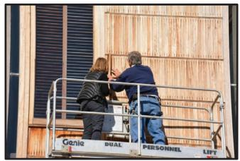
Figure 3.6. Slat removal for species identification and analysis of wood deterioration.
