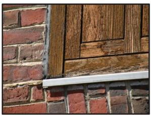
**Figure 7.12.** Close-up of teak fenestration unit on south elevation showing that the treatment has weathered severely and has been largely ineffective in maintaining the appearance or protecting the wood.
