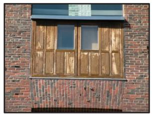
Figure 7.11. Third floor, teak fenestration unit, south elevation.
